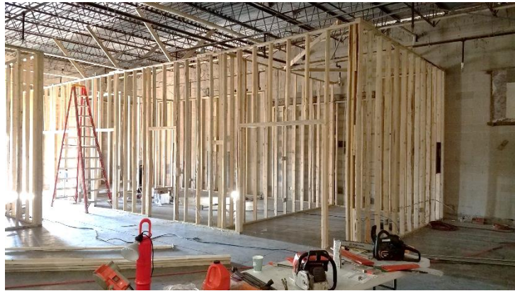
Construction at Riverside Community Church warehouse
